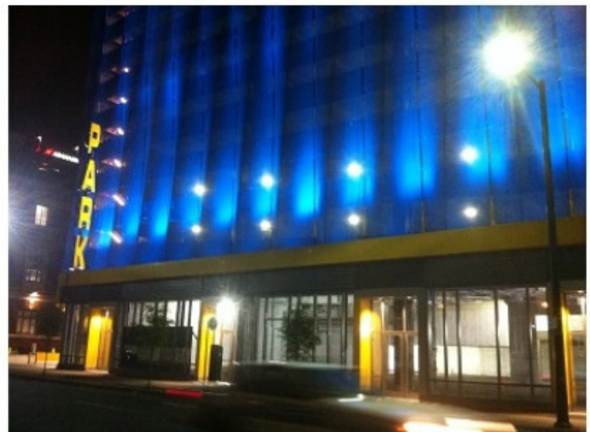
*ACTUAL PICTURE OF PARKING GARAGE*
